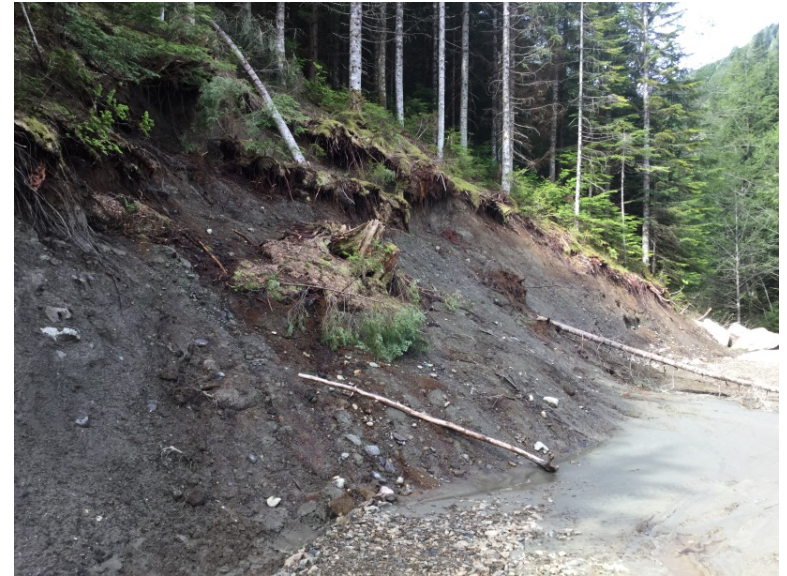
Cut slope at right approach
