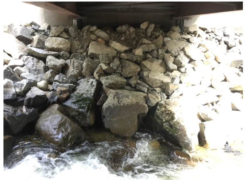
Left Bank Abutment when facing downstream
