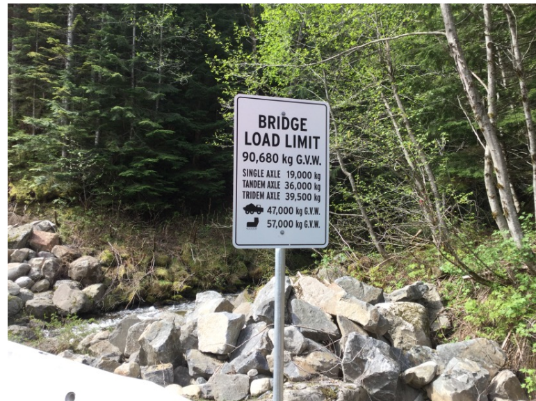
Load Rating Sign
