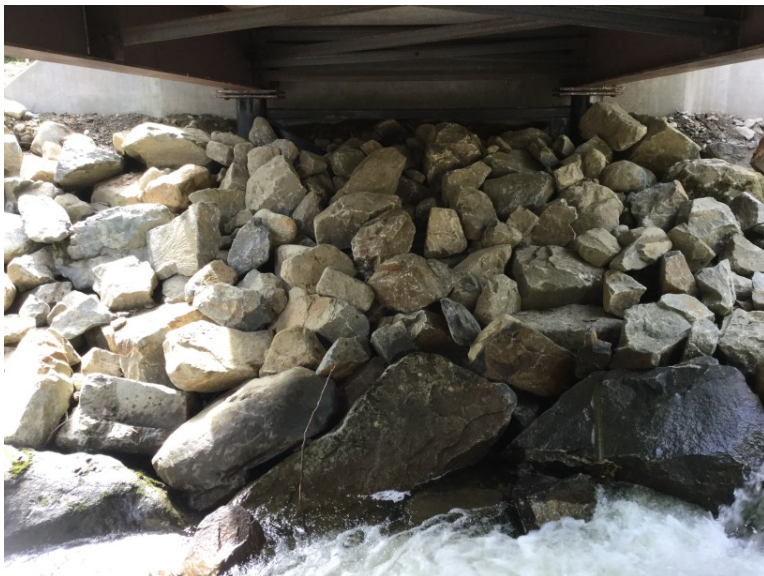
Right Bank Abutment when facing downstream
